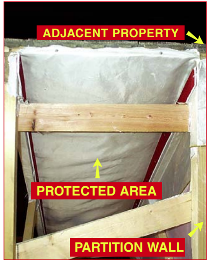
BEFORE THE FIRE TEST
